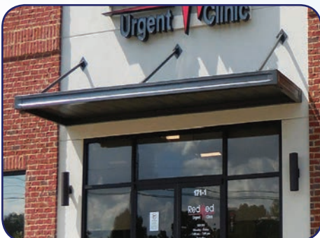
Roll Form Fascia On Entrance Canopy
