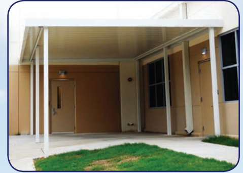
Metal Canopy With Flat Pan Decking
