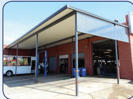
Canopy Using Roll Form Fascia & Decking
