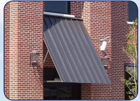
Entrance Awning With Open Ends
